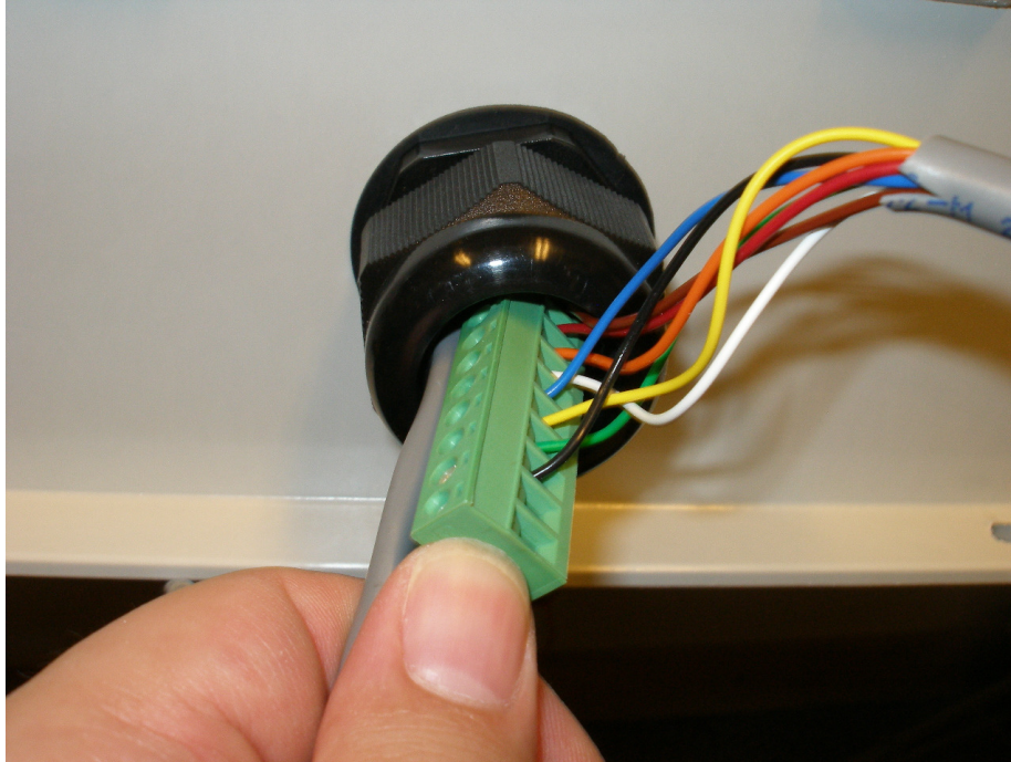
Fig 1.7 Passing the green pluggable terminal through the cable gland
